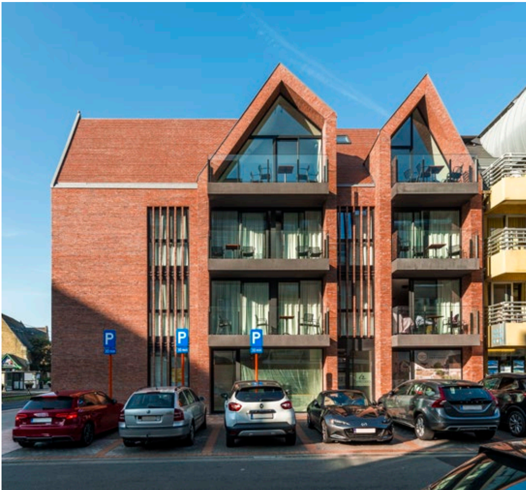
Gevel: Terca Metropolis Aula Rood Eco-brick. Dak: Koramic Tegelpan Aleonard Pontigny Vieilli naturel
