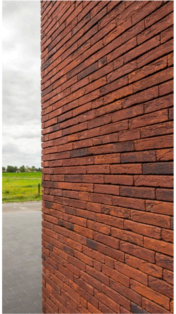
Architectenburo Acke-Van Wynsberghe, Assenede
