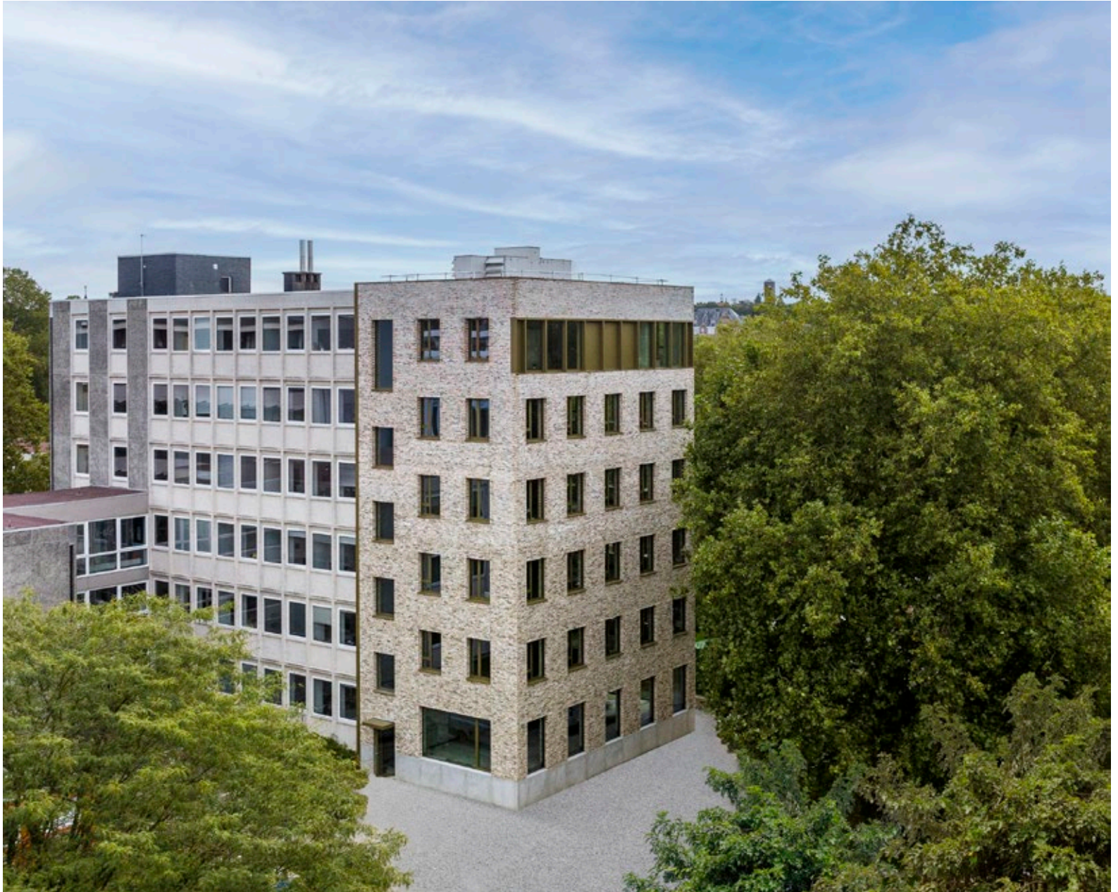
KU Leuven applied ClickBrick Pure Brons Rustic in a circular pilot project, the extension of a research building for the Department of Mathematics.
