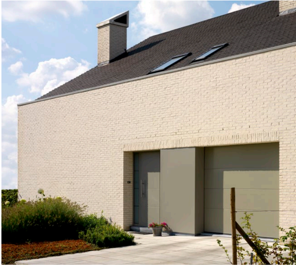
Terca Agora Superwit Architect Ignace Gheysens, Lauwe
