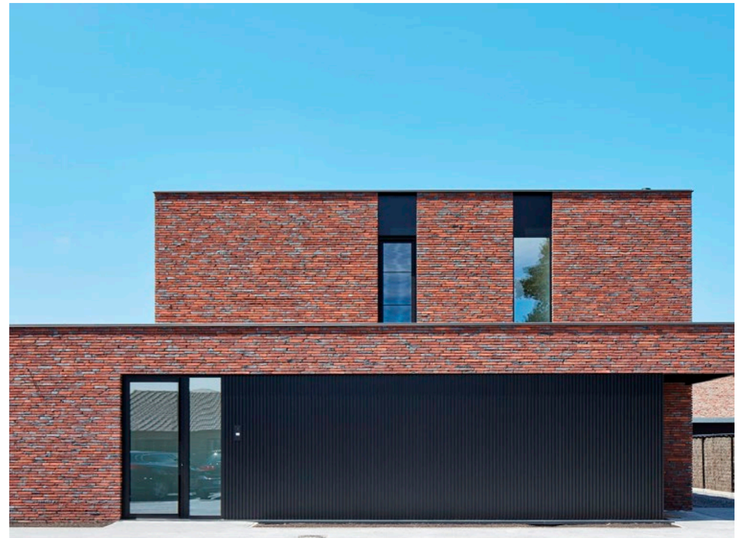
Brick-mix van Terca Linaqua Vino en Linaqua Viola studio segers architecten, Maaseik
